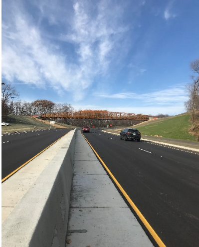
Looking north on Highway 101 open to traffic.
