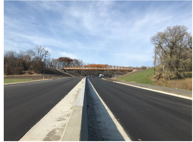
Highway 101 looking north from Highway 61 with bituminous paving complete.
