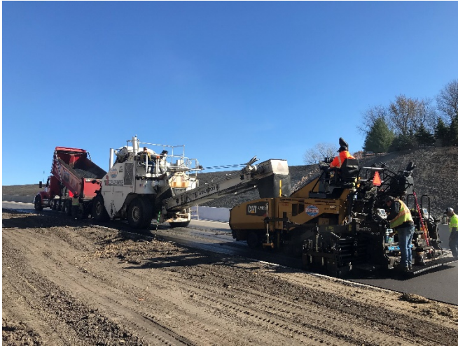
Final bituminous paving on Highway 101.
