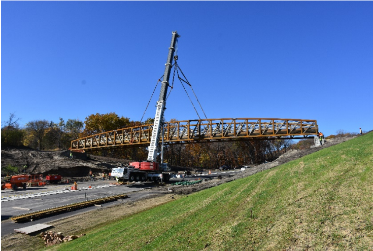
HCRA Trail Bridge placement.
