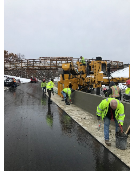
Concrete median barrier construction on Highway 101.
