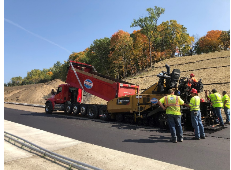
Bituminous paving on Highway 101
