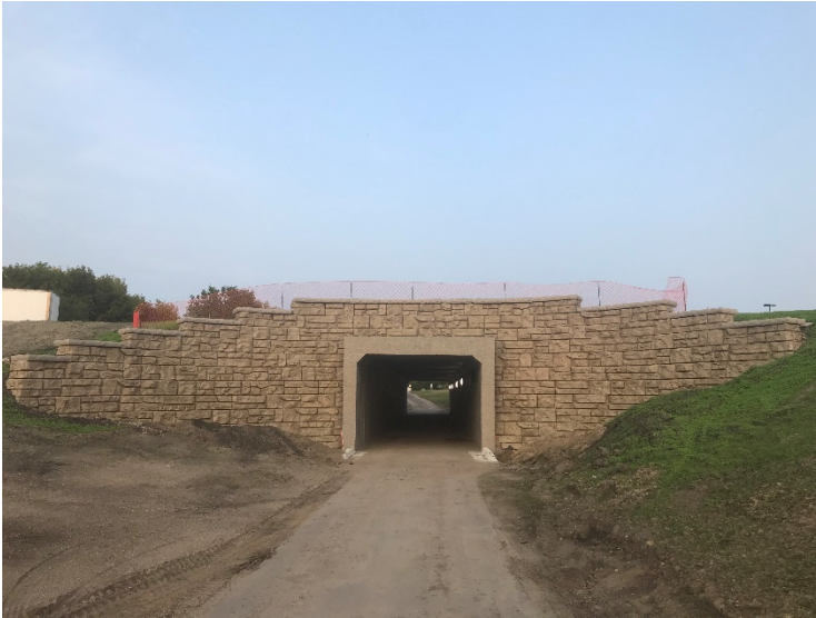
Pedestrian underpass at Highway 101 north of the Highway 61 roundabout
