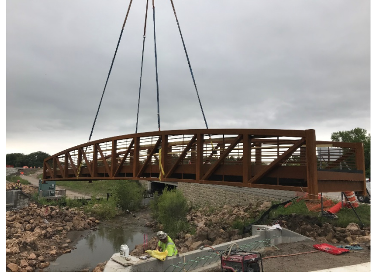
Placement of the pedestrian bridge over Bluff Creek
