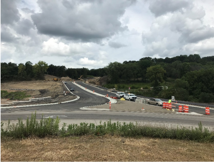
Highway 101 looking north from the Highway 61 roundabout
