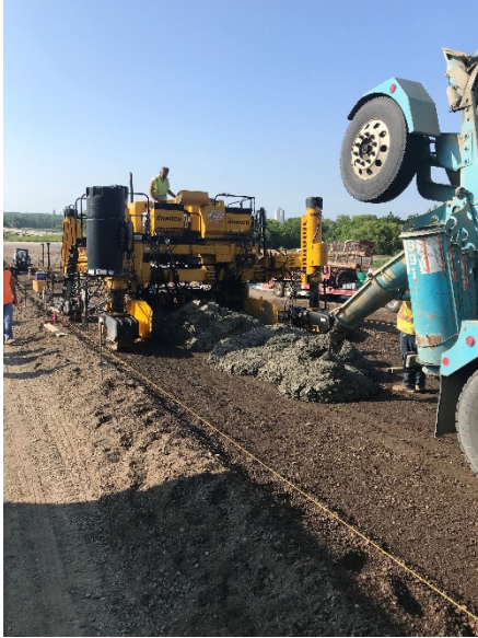
Concrete median construction along Highway 101
