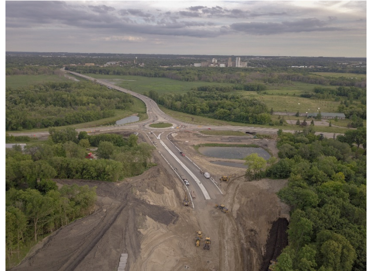
Aerial image of Highway 101 construction looking south at the Highway 61 roundabout
