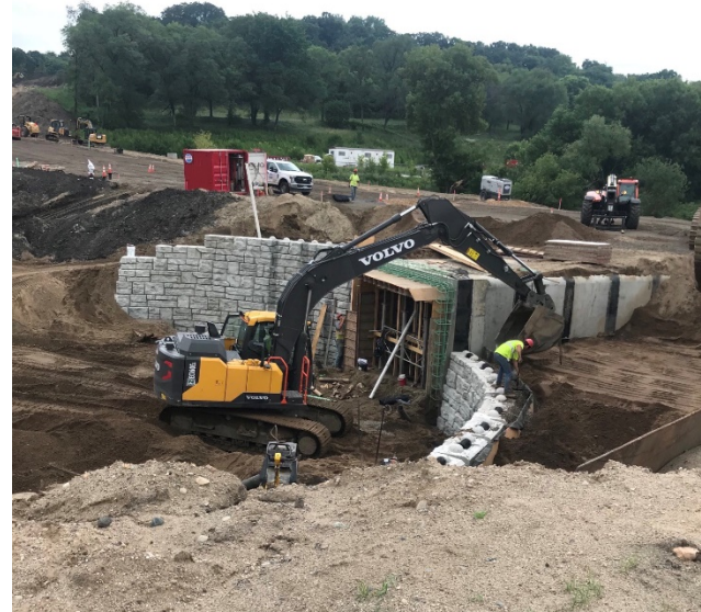
Retaining wall construction at the box culvert pedestrian underpass
