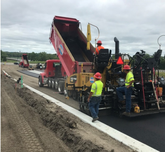
Bituminous paving along a portion of Highway 101
