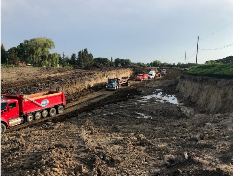
Excavation and grading activities along Highway 101
