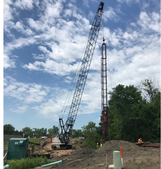
Pile driving operations for the Bluff Creek pedestrian bridge
