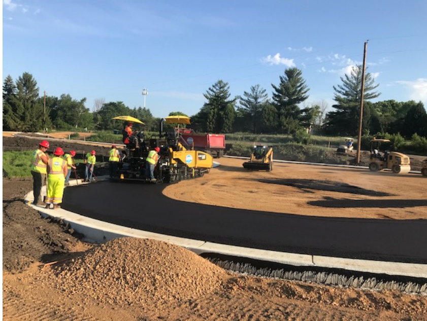
Bituminous paving on the Creekwood Drive cul de sac
