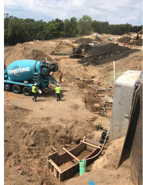
Retaining wall construction at the Highway 101 box culvert pedestrian underpass
