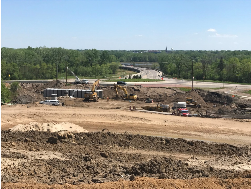
Grading and box culvert work looking south at the Highway 61 roundabout
